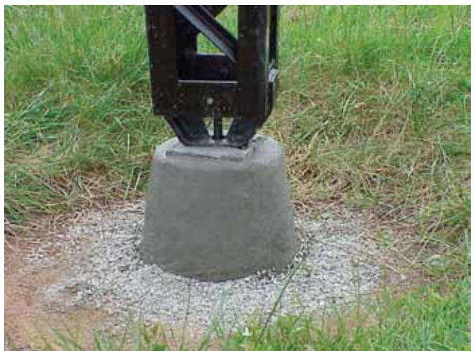
The photos show a broken foundation found during inspection (left) and a repaired foundation with a ground line coating (right). Photo courtesy of Alan Holloman, Georgia Power Co.
