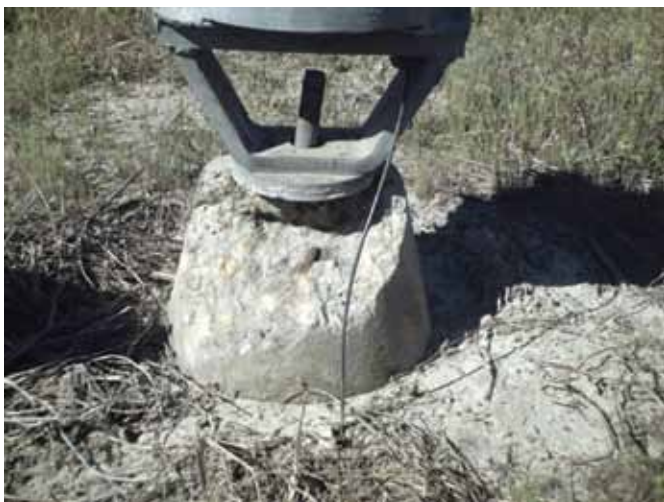
The photos show a broken foundation found during inspection (left) and a repaired foundation with a ground line coating (right). Photo courtesy of Alan Holloman, Georgia Power Co.
